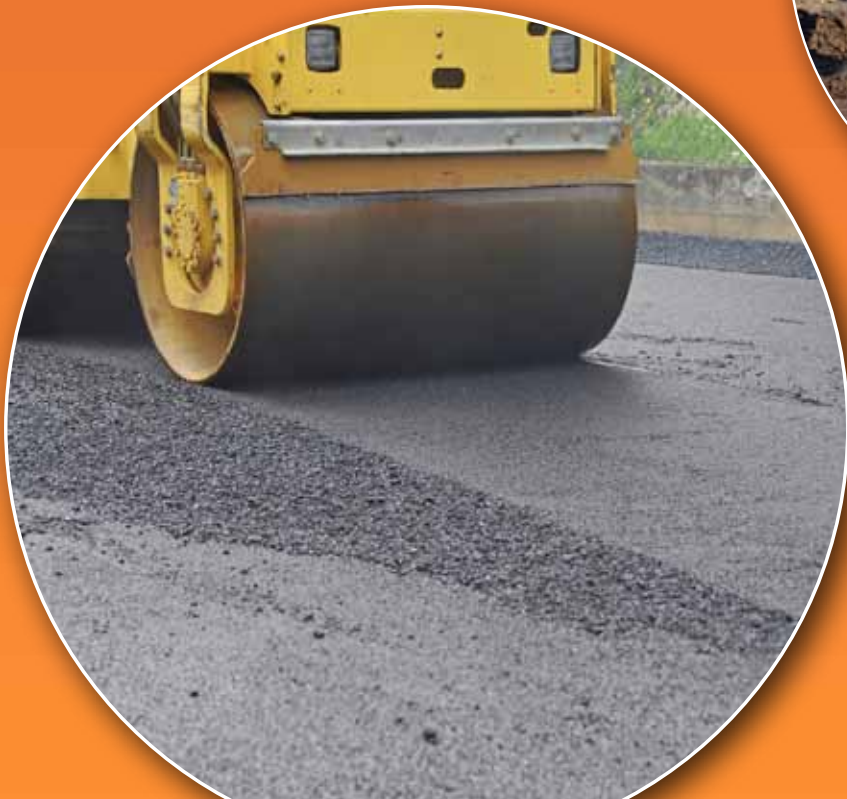
Civil & Road Building
